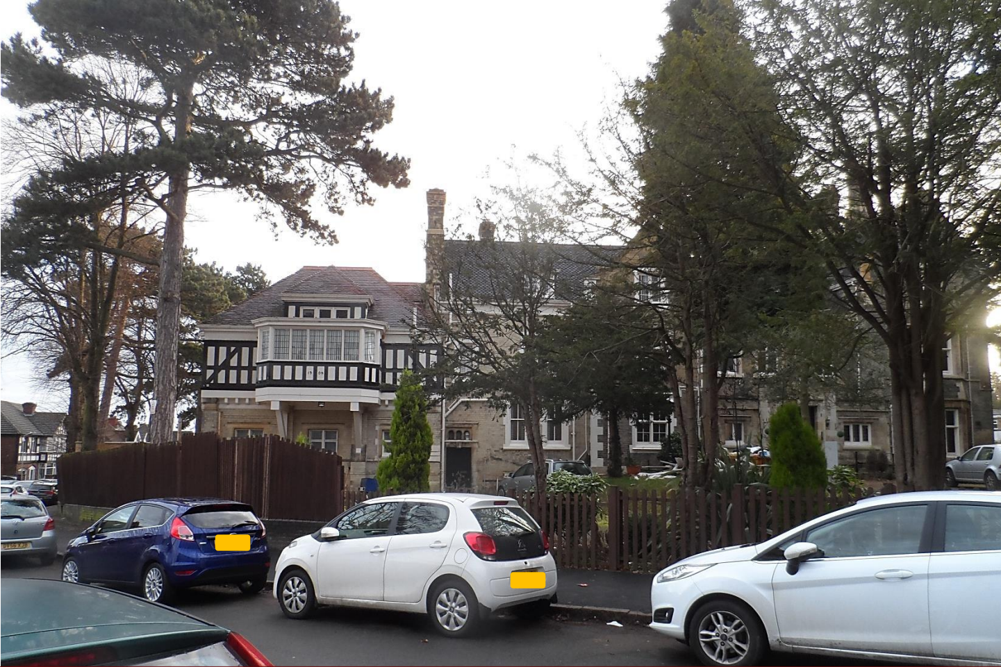
Front of building
